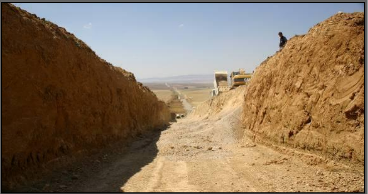
Bedding after ground stabilization
